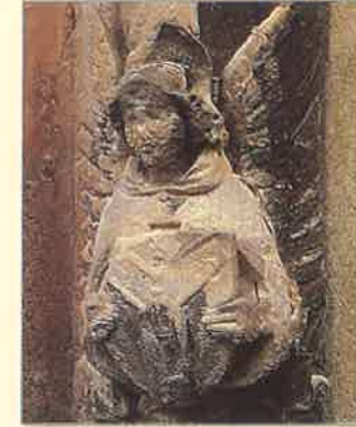
Many buildings are being destroyed by acid rain.
