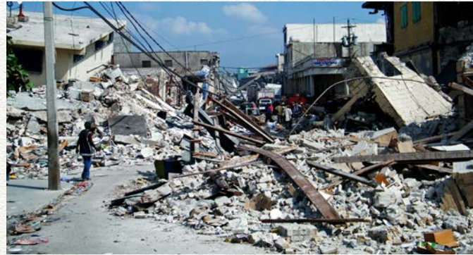
Severe damage occurred during the earthquake in Haiti in 2010.
