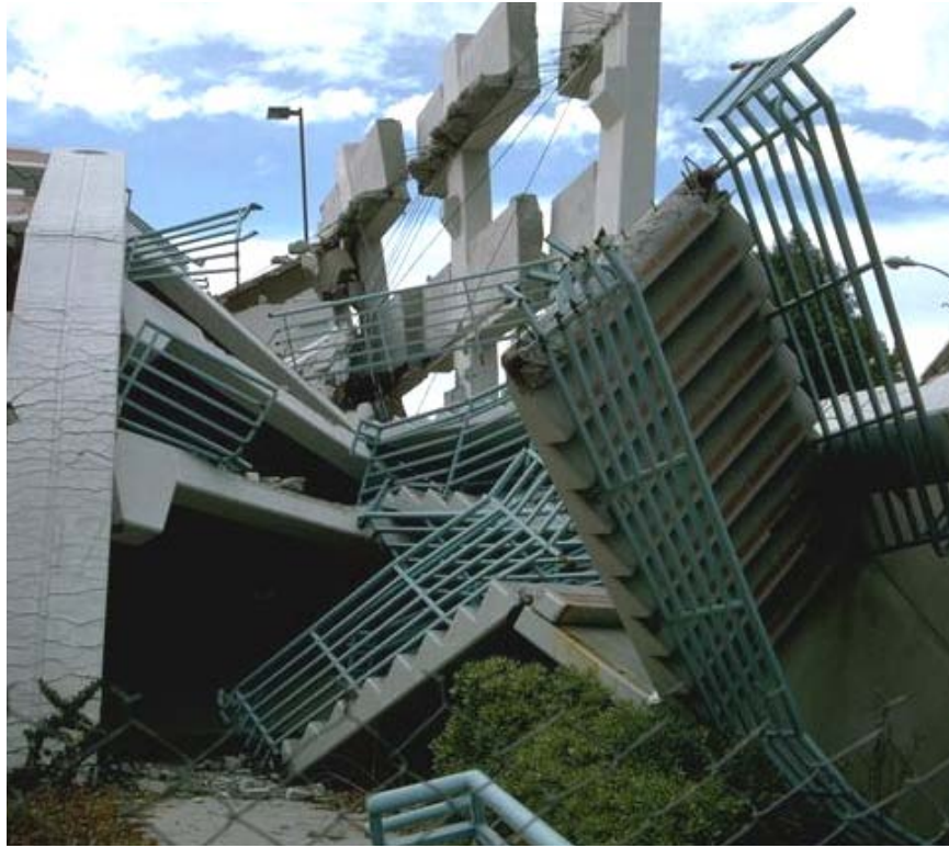
An earthquake destroyed this building.
