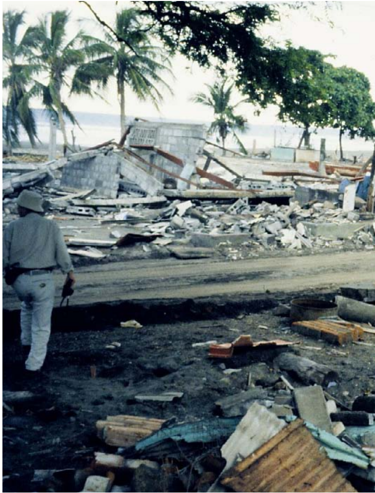
Damage from a tsunami
